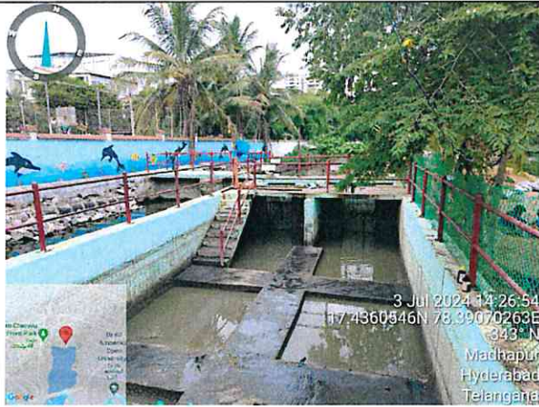
Durgam Cheruvu interception and diversion structure
