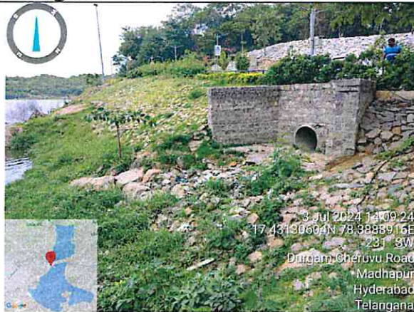
Durgam Cheruvu storm water drain inlets
