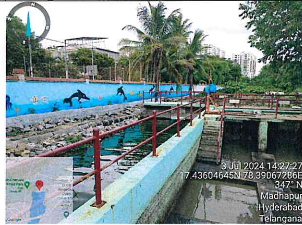
Durgam Cheruvu interception and diversion structure
