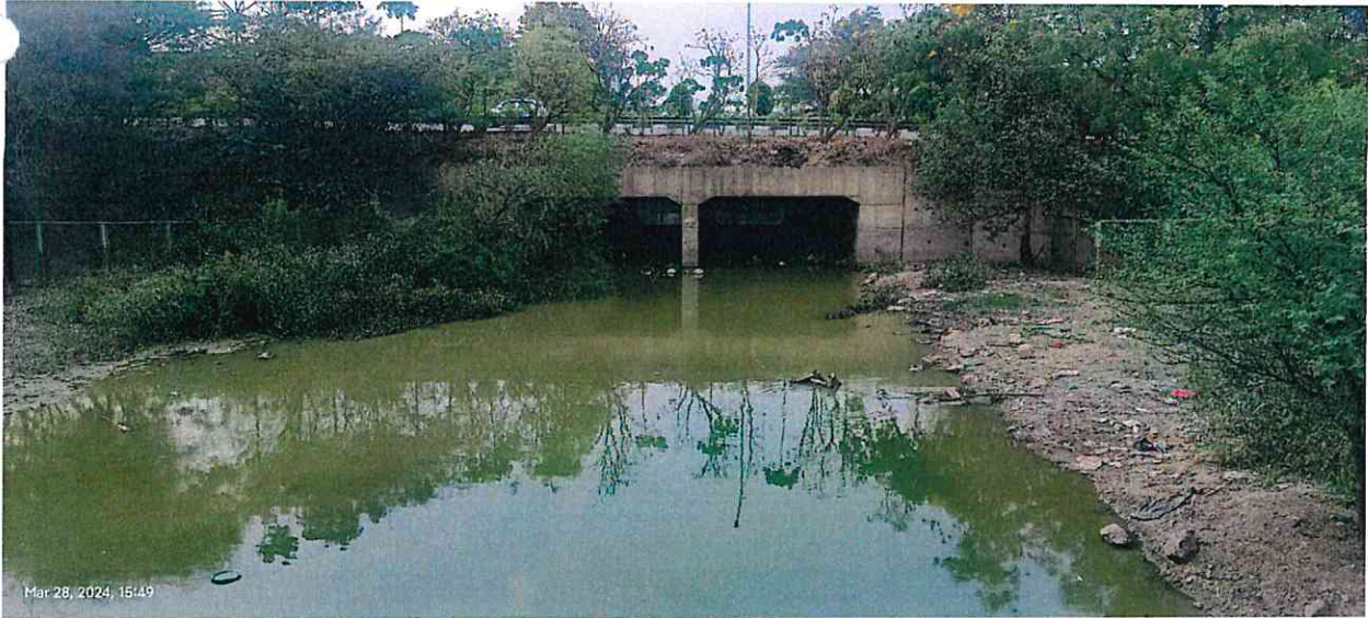
Inlet drain joining into Chinnadamara cheruvu near ORR service Road
