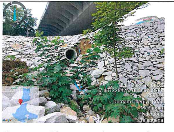
Durgam Cheruvu storm water drain inlets
