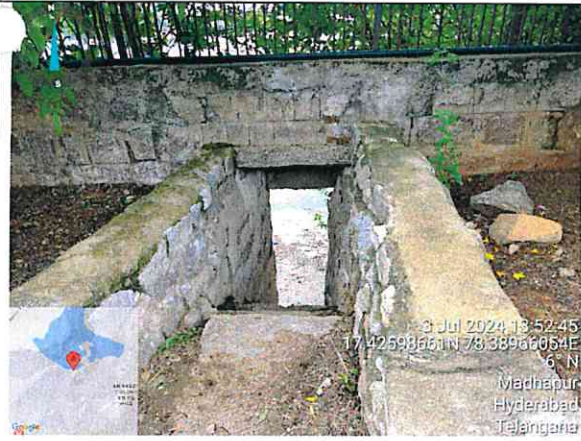
Durgam Cheruvu sluice area
