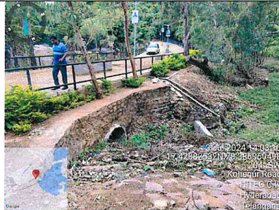
Durgam Cheruvu storm water drain inlets
